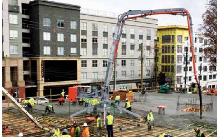
Above: All eight 310-foot by 180-foot floors of the structure are being pumped through one Spider Boom.
