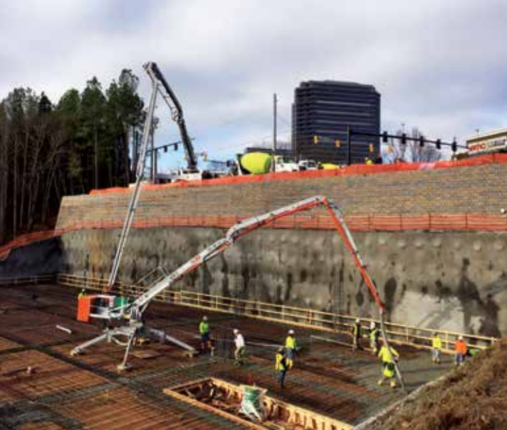
Above: All eight 310-foot by 180-foot floors of the structure are being pumped through one Spider Boom.
