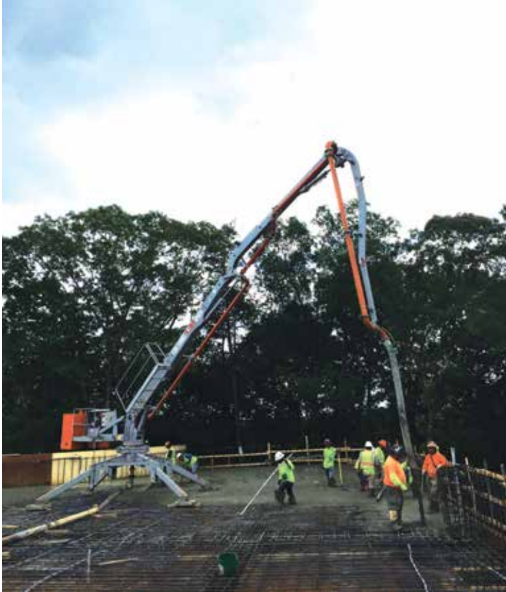
The smooth boom operation and balanced design with counterweight allows the Spider Boom to operate without being tied down to the deck.
